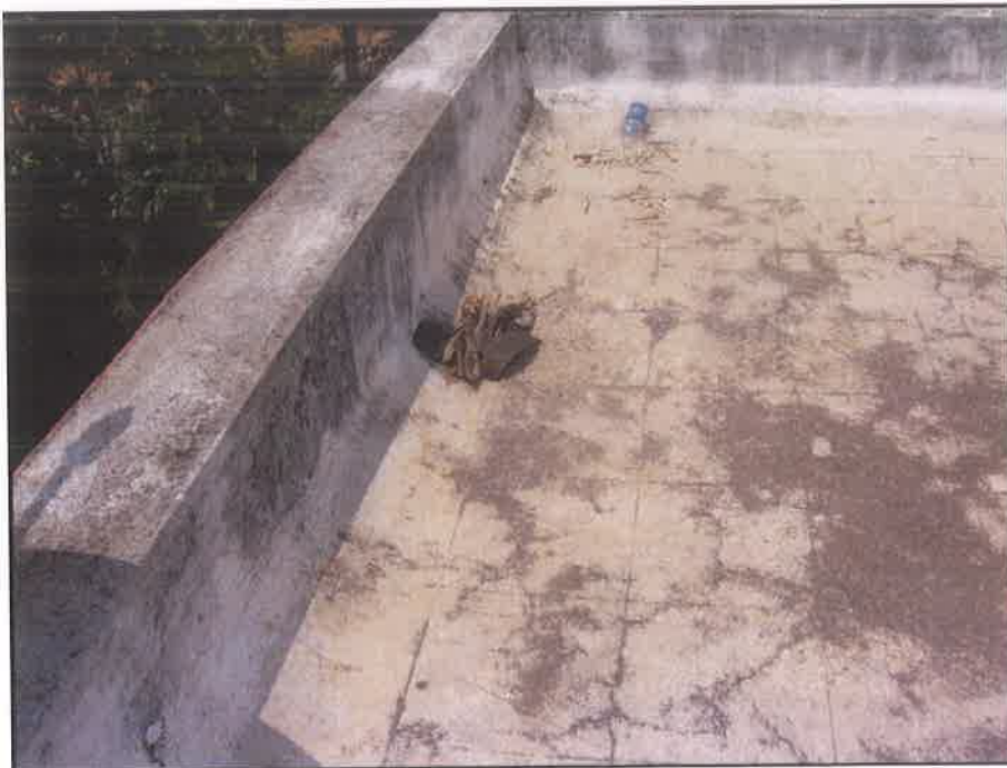
Chocking of rain water outlet (Typical views)
