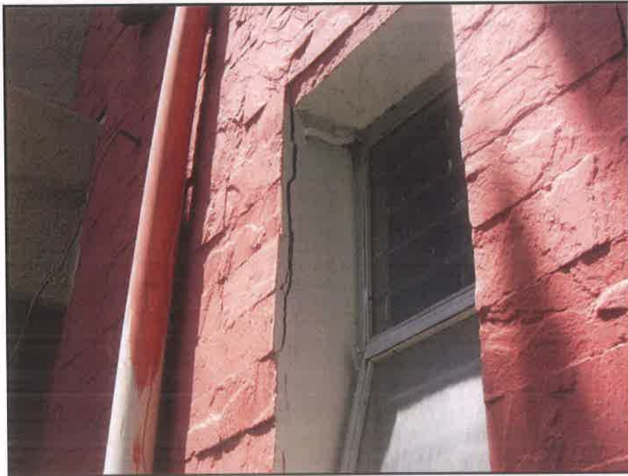
Debonding of cladded tiles
