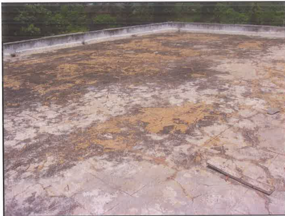
Crack in WPC over roof slab
