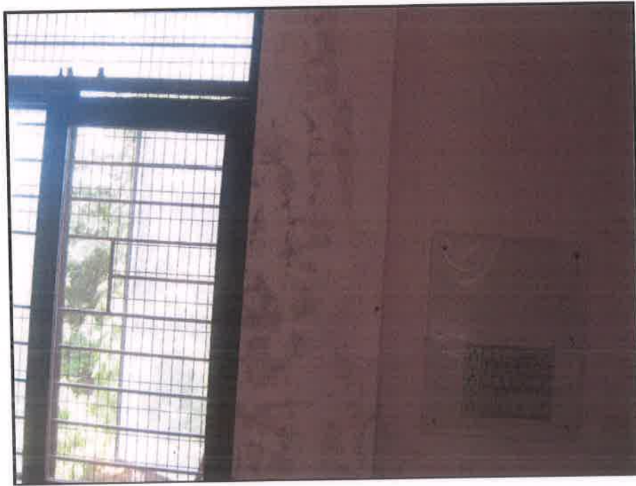
Damp patches in RC column and ceiling slab
