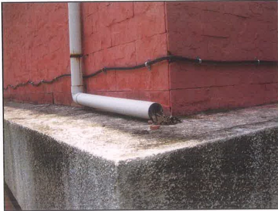
Chocking of rain water outlet (Typical views)
