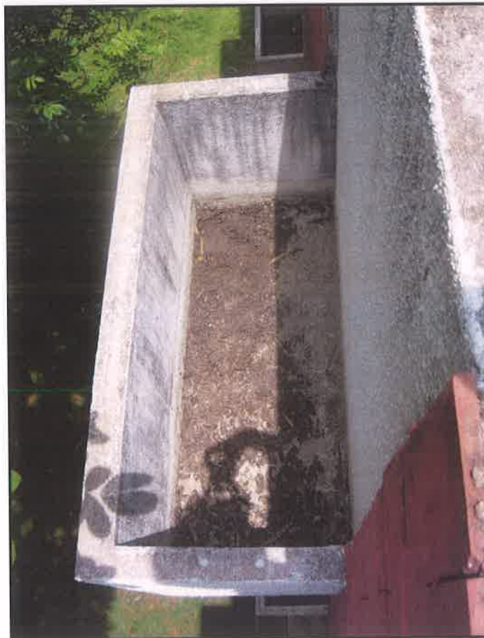
Accumulation of waste materials over chejja
