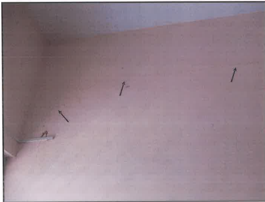
Separation crack between masonry wall and RC members
